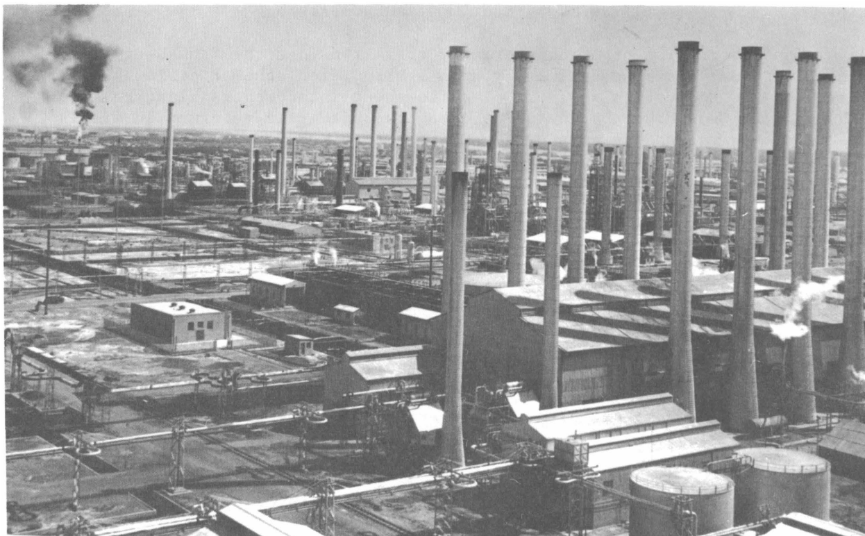
FIGURE 22. - General View of Abadan Refinery Looking Almost Due South From the Vicinity of the Catalytic Cracking Unit. Special products area boilers are in right foreground, and flare area is in left middle background.
