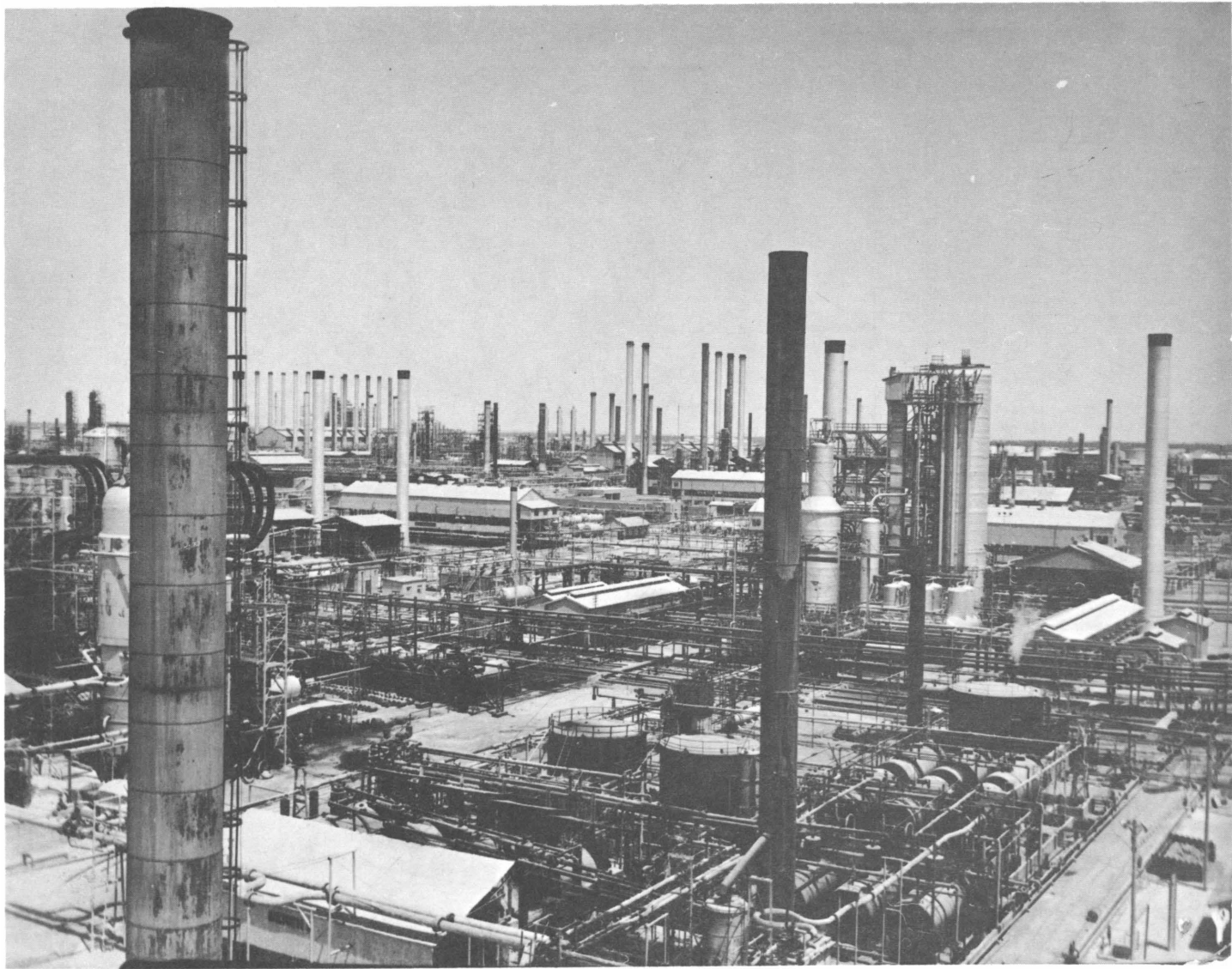
FIGURE 21. - General View of Abadan Refinery Looking Almost Due North From the Crude Oil and Bitumen Distillation Area. One of the primary distillation towers can be seen to the right of the black stack in the foreground. The catalytic cracking tower is on the horizon behind the left group of stacks. (Courtesy of NIOC.)
