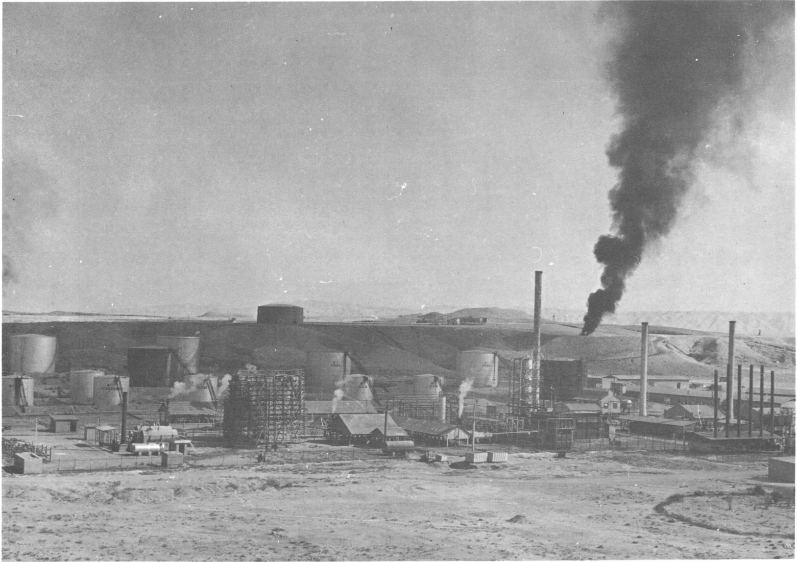
FIGURE 26. - NIOC's Naft-e Shah Topping Plant in Western Iran. (Courtesy of NIOC.)
