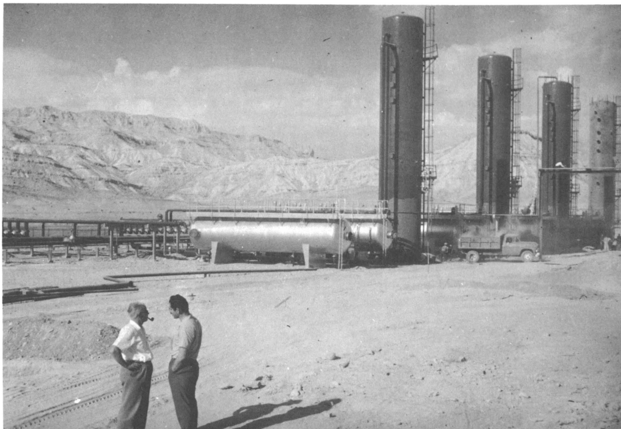
FIGURE 10. - Production Unit No. 3, Gach Saran, Under Construction.
