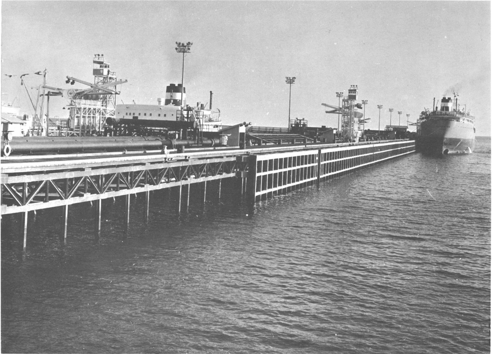
FIGURE 30. - Jetty at Kharg Island. (Courtesy of NIOC.)
