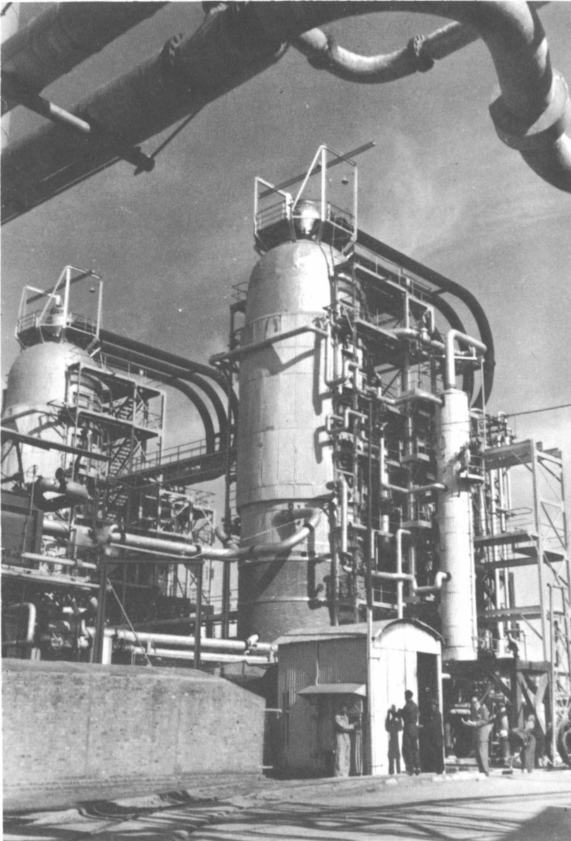
FIGURE 24. - Primary Crude Distillation Tower at the Abadan Refinery.
